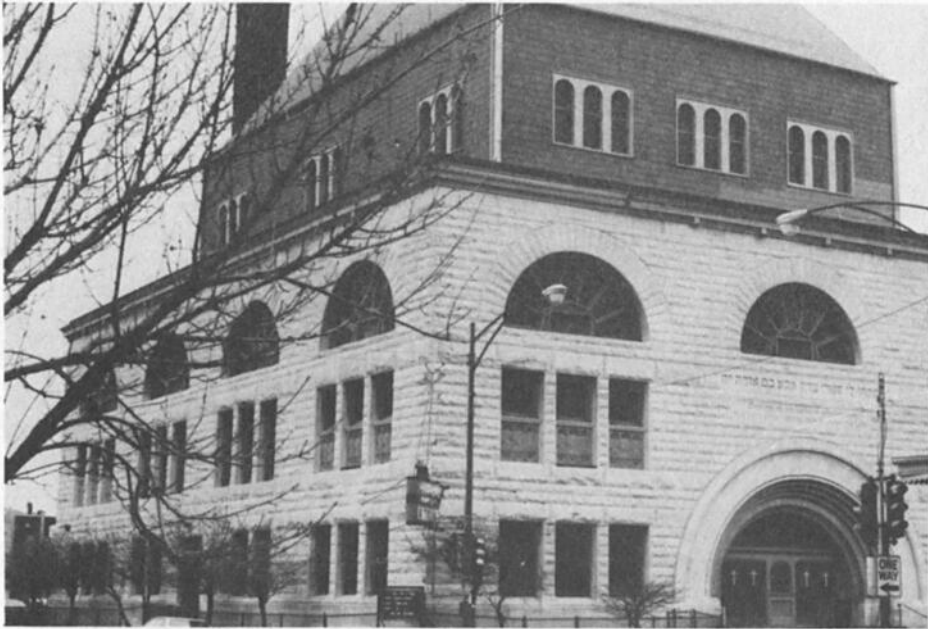
Chicago's K. A. M. ("Congregation of the People of the West") built this synagogue in 1890-91. Designed by Dankmar Adler and Louis Sullivan, it is one of the few American religious structures built in the Chicago School style of architecture. The building is now a designated city landmark and a Baptist church.
